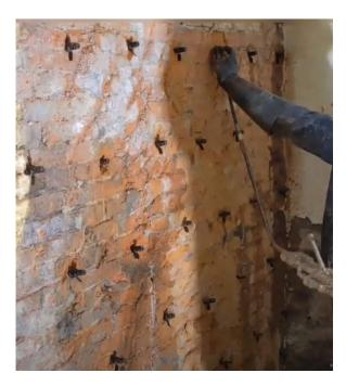
Figure 33. System involving injections of acrylic resins
