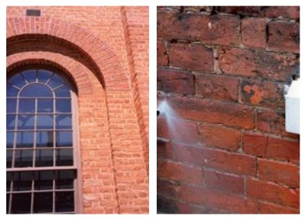
Figure 32. Abrasive (left) and chemical (right) cleaning techniques
